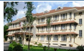
NIHE High Tech Build.
