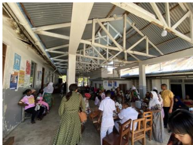
Bagamoyo District Hospital
