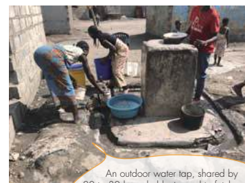
An outdoor water tap, shared by 20 to 30 households, is used to fetch water. The faucet is located right on the ground due to the low water pressure. Water is stored at home, but contamination occurs by the time it is consumed.
