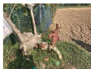
Pump drawing up arsenic-containing groundwater for irrigation
