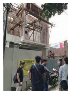
Inspection of a masonry house construction site
